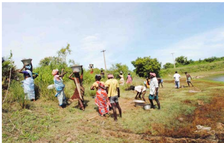
Rejuvenation of Pond
