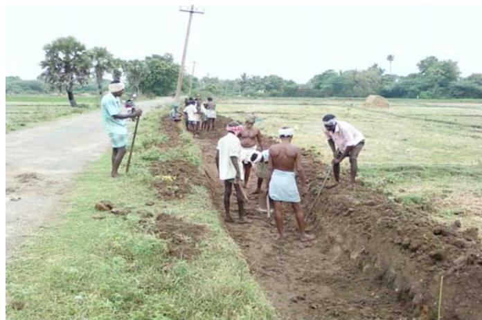
Renovation of Irrigation Channel
