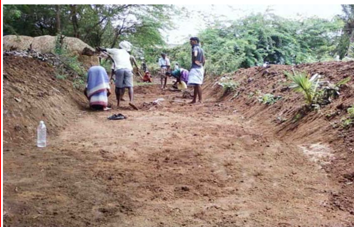
Supply Excavation Channel
